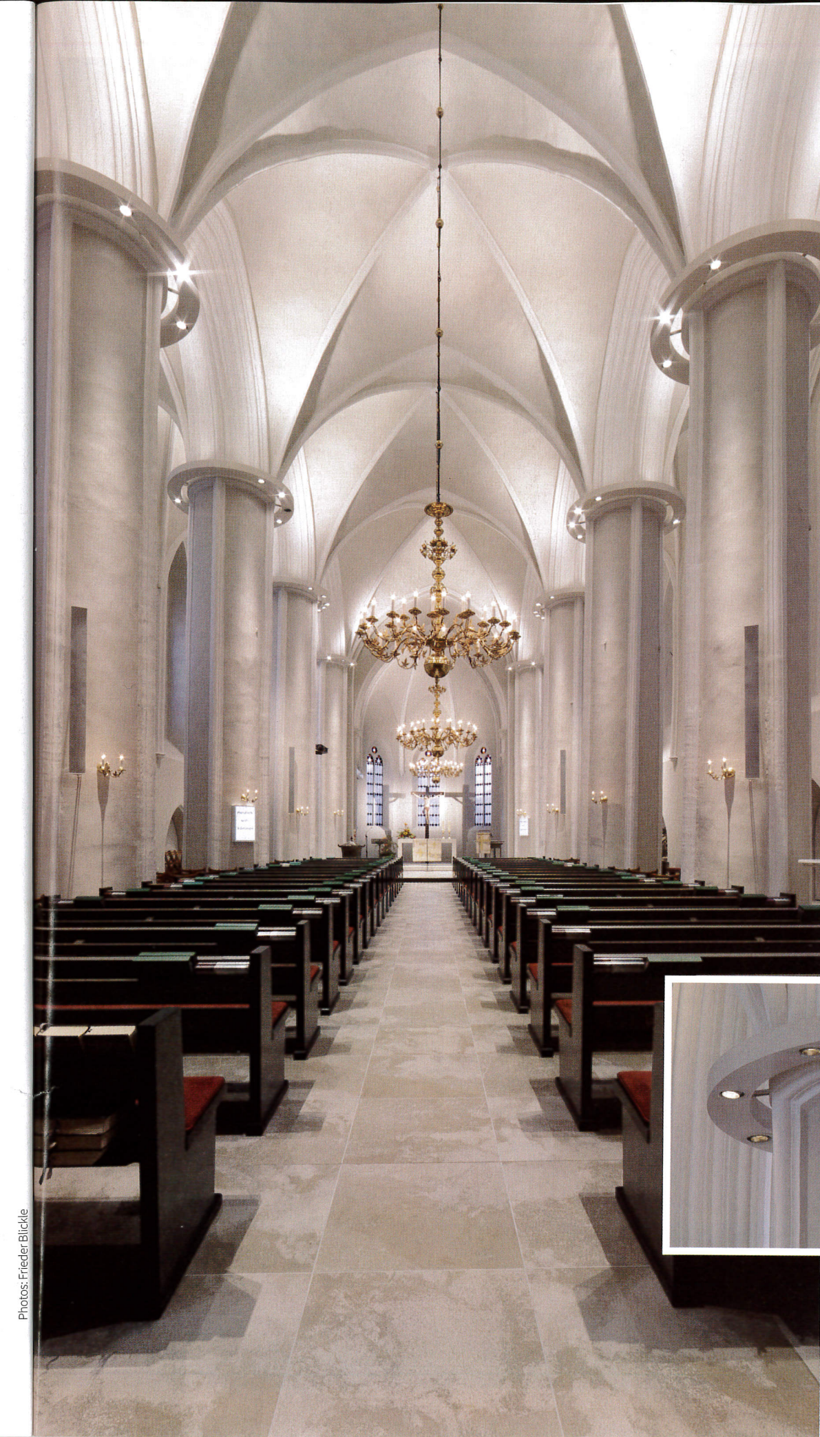
Luminaire rings surrounding each pillar proved to be a minimally invasive design solution for the first millennium church. Restored chandeliers add to the ambient light.
